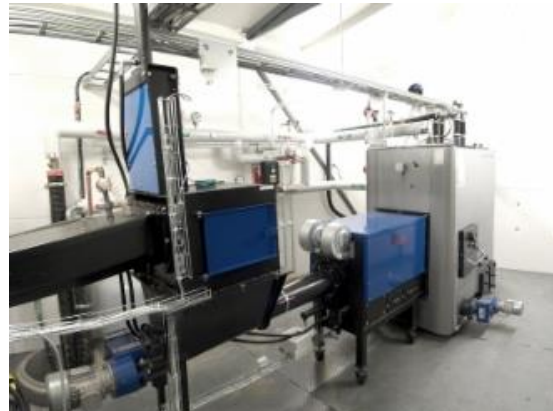
IMAGE 9. Wood-chip heating container 60-500 kW ( http://www.biofire.fi )
